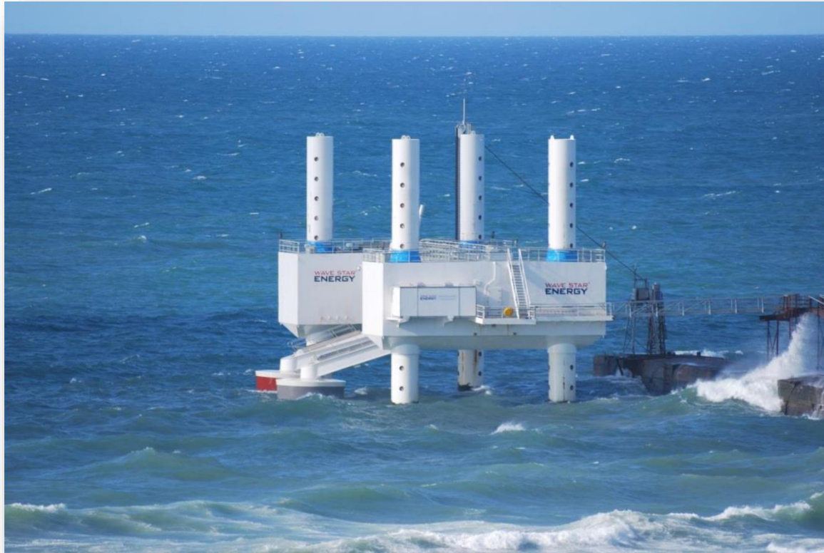
Wave Star wave energy generator located at the Hanstholm test site in Denmark. (Courtesy of Wave Star Company.)
